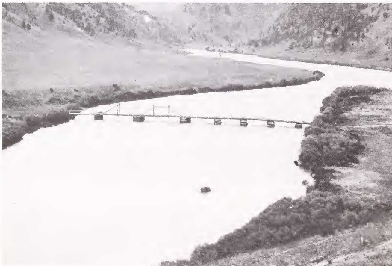
The Scanland Toll Bridge on the Madison River, Circa 1871. (W. H. Jackson Collection, Museum of the Rockies).
